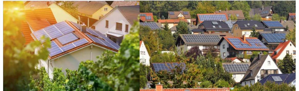
Ost-West-Installation © Trifilat
