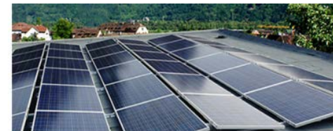
Ost-West-Installation © Trifilat
